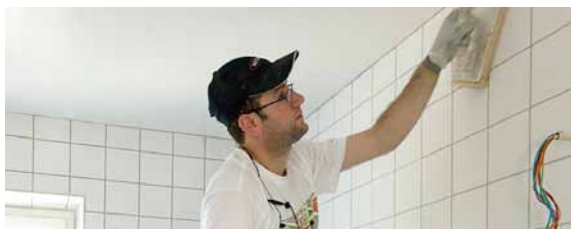
New tiles are being laid in a bathroom, which is being fully renovated in conjunction with the replacement of central plumbing.
